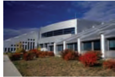
Solar Energy Research Facility at NREL
